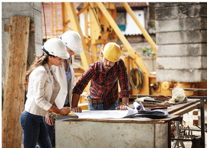
On a construction site
